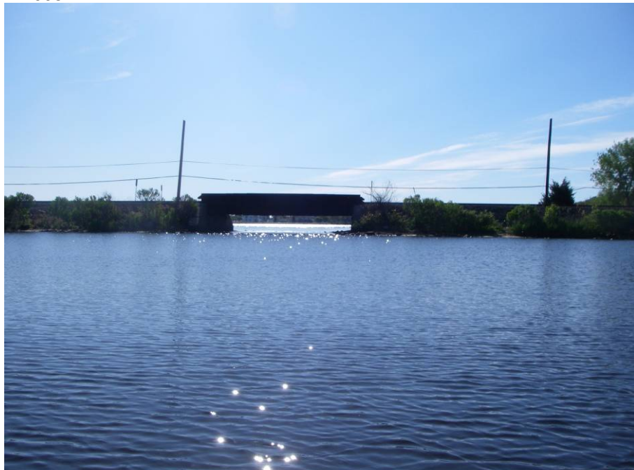
Photo 2: View facing east towards the New Jersey Transit railroad bridge and fyke net location. Photo taken in 2008.
