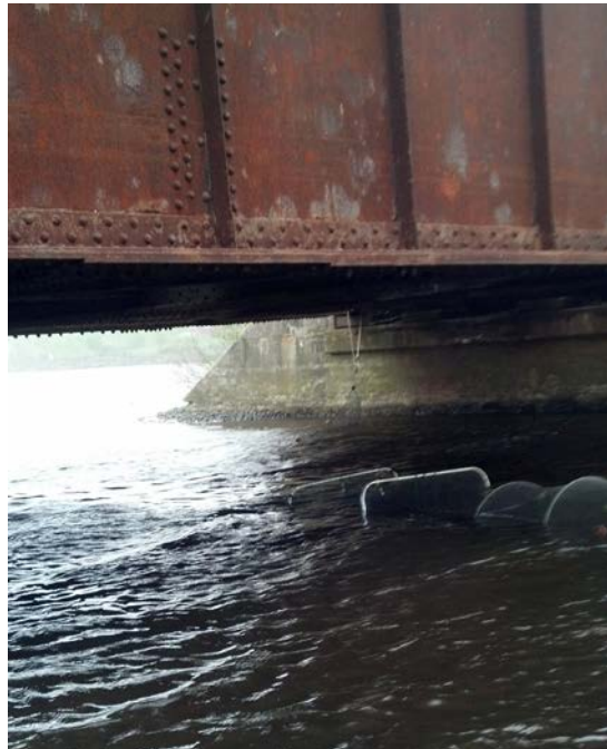
Photo 4: Net set under railroad bridge showing centralized location and how wing was secured to the structure. Photo taken in 2014 during Sampling Event 1.
