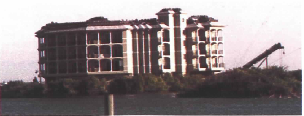
A condominium under construction on the Indian River Lagoon, Melbourne, FL.
