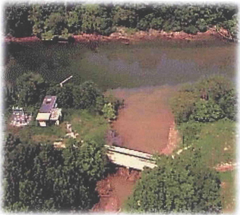
Sediment from a construction site flows into receiving waters if not properly handled.
