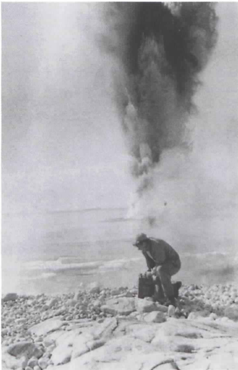
Clearing ice from the landing ship channel with explosives.
