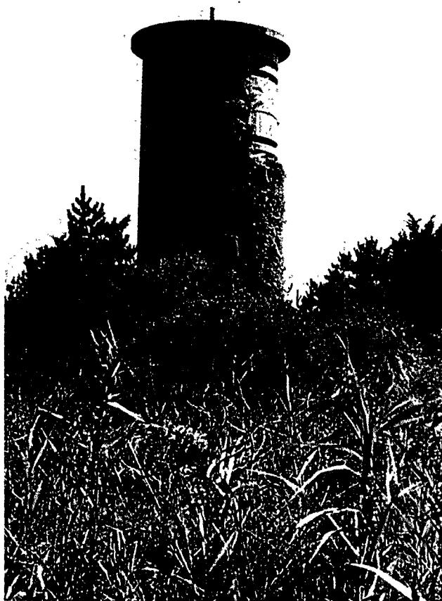
This tower, and others like it, dot the coast of southern Delaware along Route 1. Built during World War II, they were used to search the Atlantic coast for enemy submarines.
