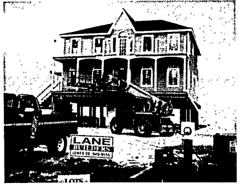
Another bayfront "McMansion;" note the ten-foot pilings used to raise the first floor above base flood elevation.
