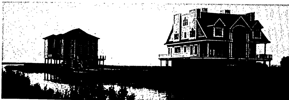
New development on Sussex County wetlands, each with 5600 square feet of "cottage" living. Water in the foreground is a man-made lagoon.
