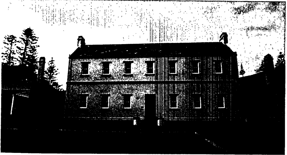
Restored military barracks on Norfolk Island.
