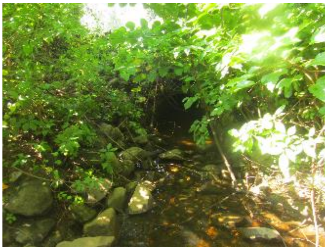
Figure 94. Culvert located at approximately GPS: 40.1467N 74.057483W.
