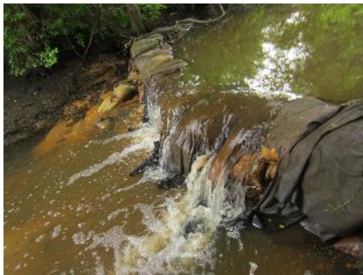
Figure 71. Sand bag weir upstream of mud flat. GPS: 40.15216N 74.09195W \pm 10' .
