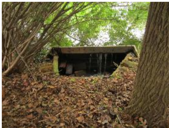
Figure 66. Impoundment upstream of Hiddenbrook Dr.
