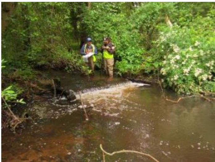
Figure 31. Wooden weir just upstream of old wooden footbridge
