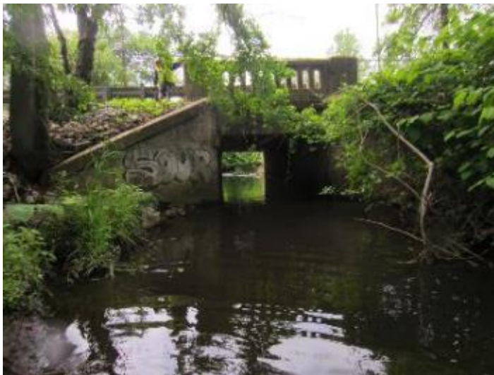
Figure 43. Route 35 Bridge/Box Culvert.
