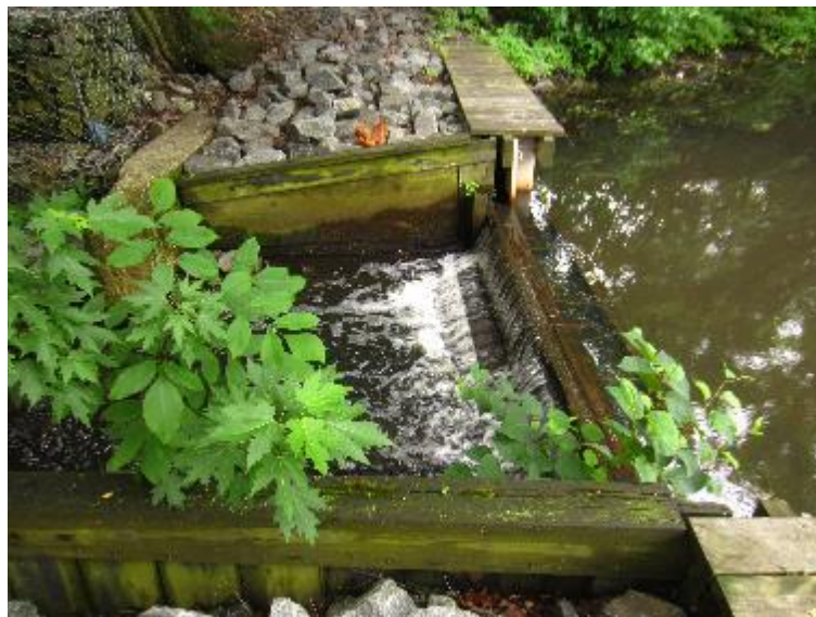
Figure 14. Weir approximately 5m upstream of Route 71 bridge.
