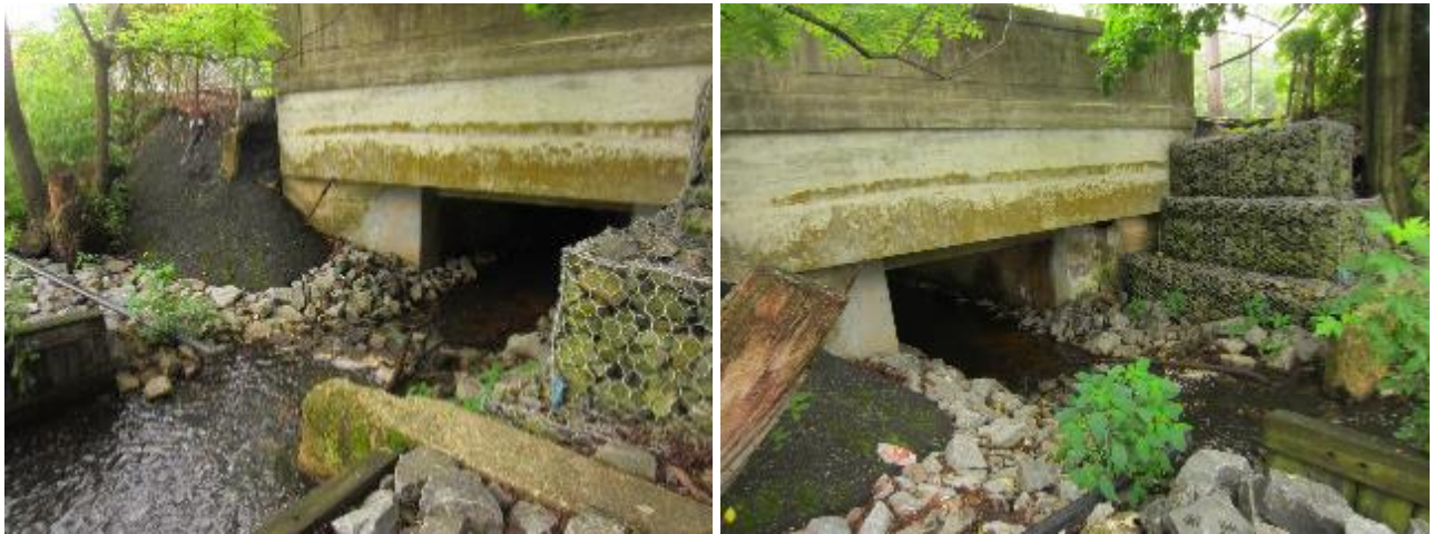
Figure 13. Upstream of the Route 71 bridge.
