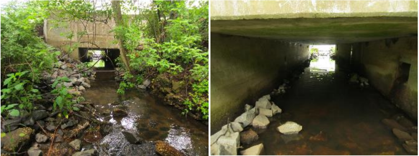
Figure 12. Just downstream and below the Route 71 bridge.
