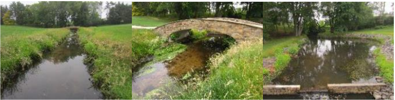
Figure 22. Upstream end of fifth pond/run and third weir.
