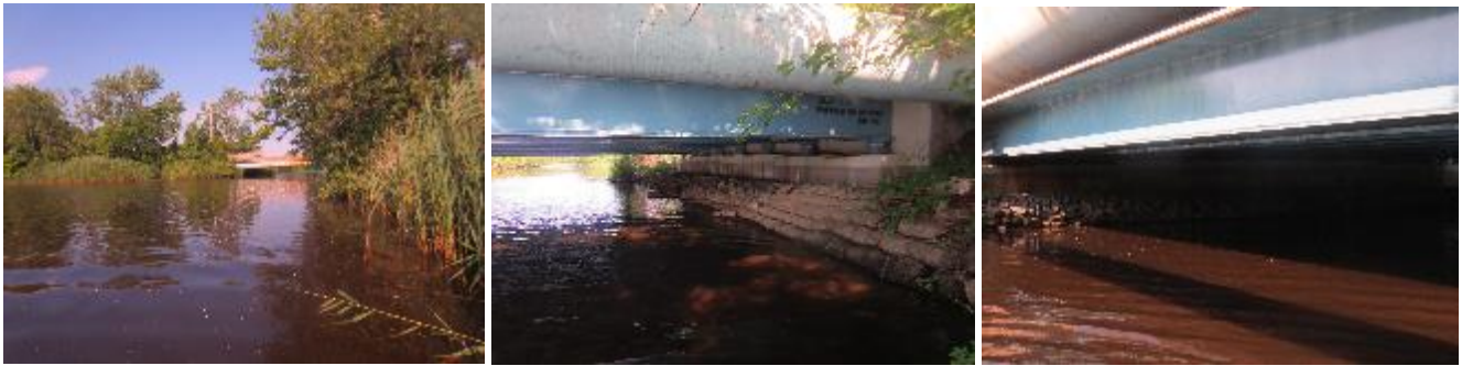
Figure 81. Route 71 Bridge, Wreck Pond.
