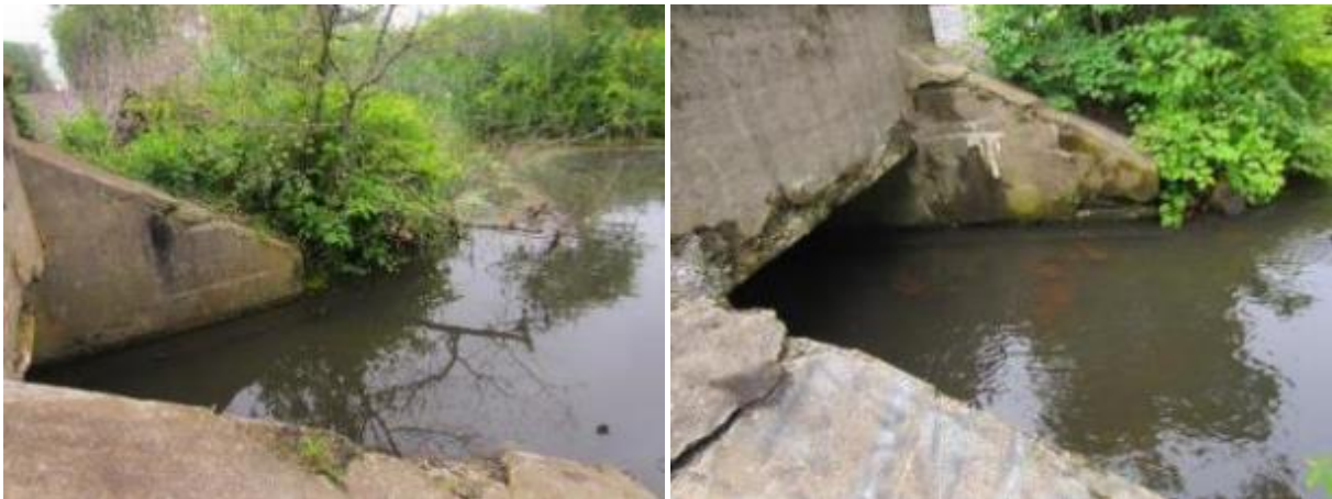
Figure 8. Downstream end of railroad (RR) bridge.
