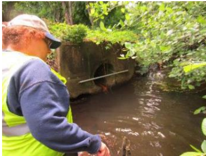
Figure 41. Concrete culvert located just upstream of stone revetment property.
