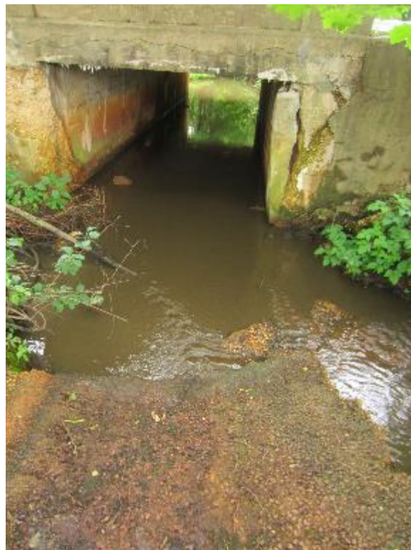
Figure 68. Culvert at Allaire Rd. Start location of June 16, 2015 survey.
