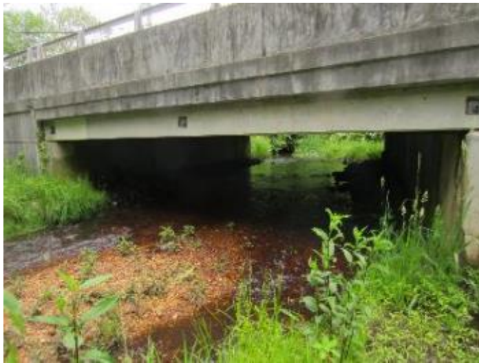
Figure 29. Old Mill Road Bridge
