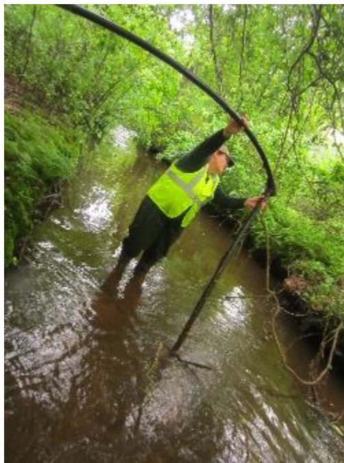
Figure 76. Long, black pipe in creek GPS: 40.14462N 74.07369W ±27'.
