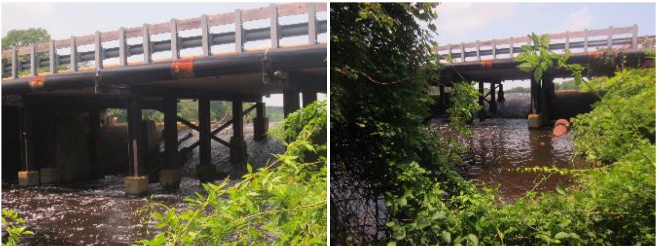
Figure 102. Wreck Pond Brook, Allaire Road Bridge and Dam. GPS: 40.15295N 74.061533W ±17'.
