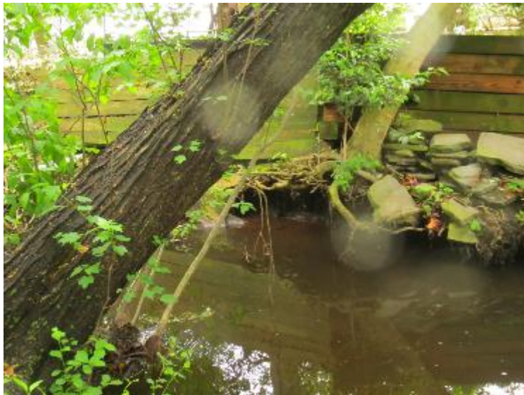
Figure 32. Undercut bank and wooden bulkhead just downstream of the Old Mill Elementary School
