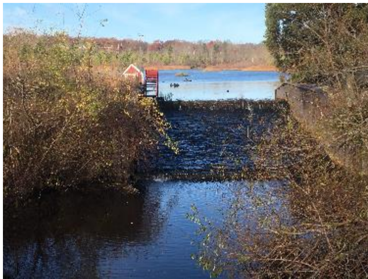
Figure 91. Old Mill Pond Dam and Old Mill Pond.
