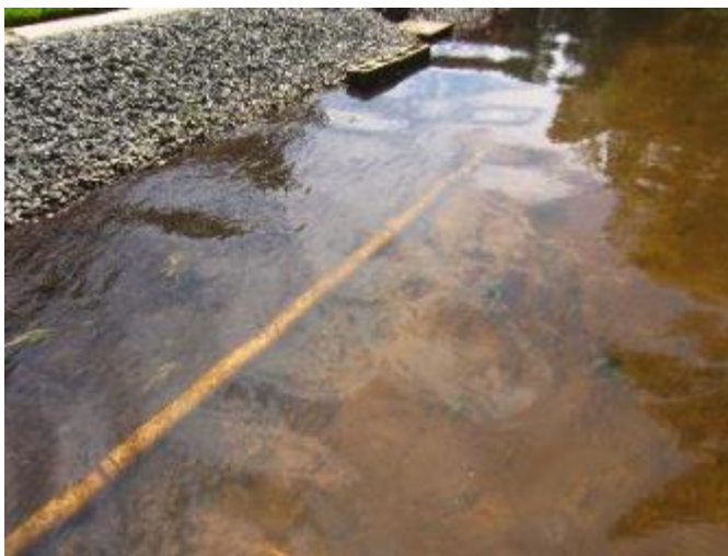
Figure 40. White, slotted pipe in creek.
