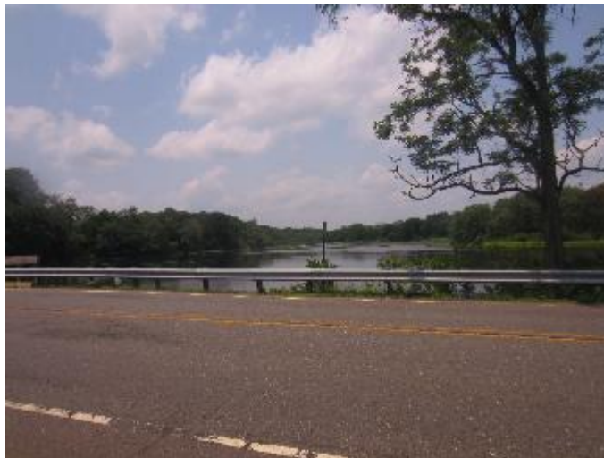
Figure 103. Osborne's Pond upstream of Allaire Road.
