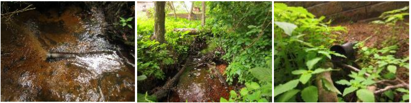
Figure 61. Black pipes emptying into creek below Crystalbrook Dr.
