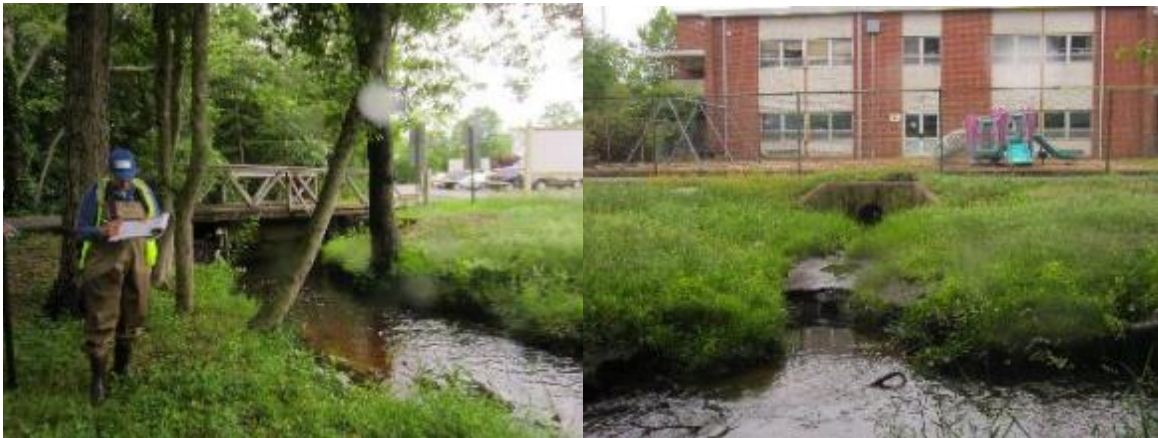
Figure 33. Footbridge and storm drain culvert at the downstream end of the Old Mill Elementary School property.
