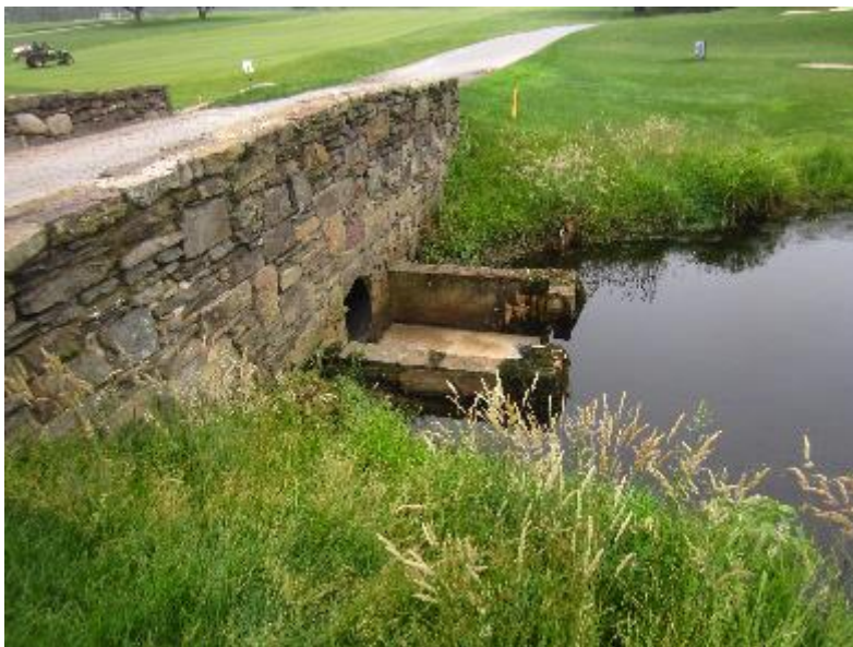
Figure 19. Culvert separating fourth pond and fifth pond/run.
