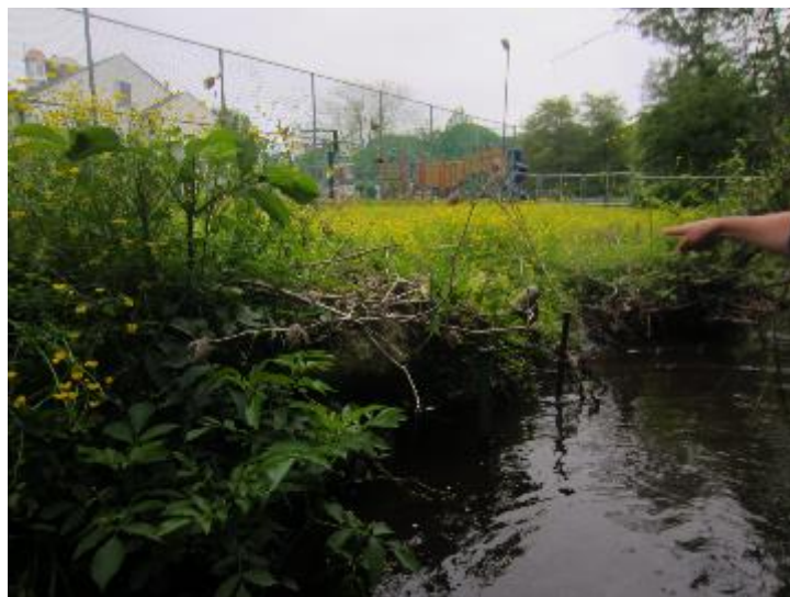
Figure 46. Small, grey pipes emptying into creek at The Brookside School.
