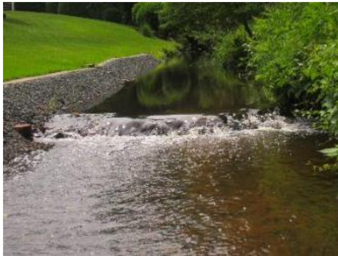
Figure 39. Small, concrete check dam located half way along residential property.
