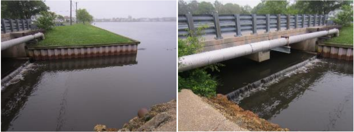
Figure 1. Black Creek Weir, downstream Wreck Pond side
