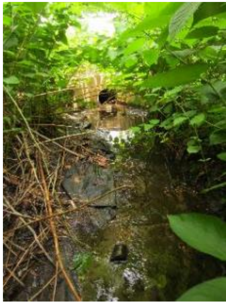
Figure 56. Culvert located approx. 5m below Bailey's Corner Rd. GPS: 40.14214N 74.06772W ±16'.
