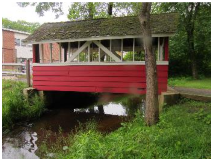
Figure 34. Second footbridge at the Old Mill Elementary School property.
