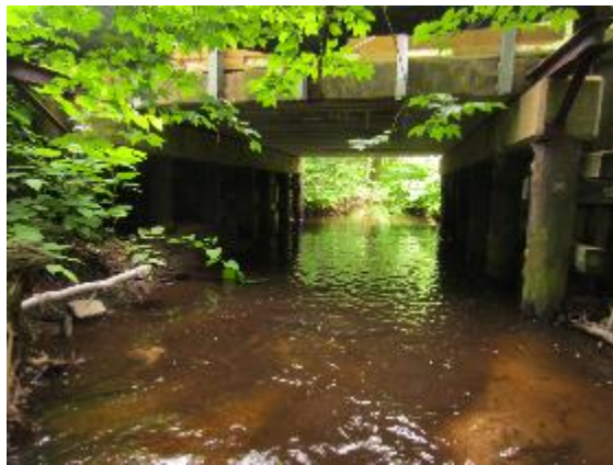
Figure 57. Looking downstream through Bridge at Bailey's Corner Rd, Hannabrand Brook.
