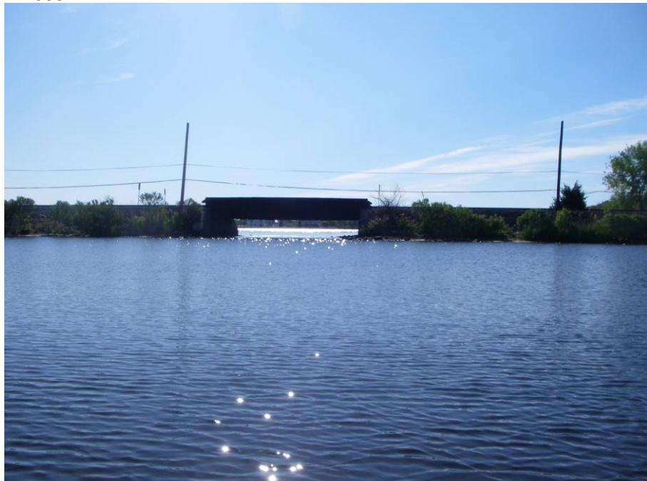
Photo 2: View facing east towards the New Jersey Transit railroad bridge and fyke net location. Photo taken in 2008.
