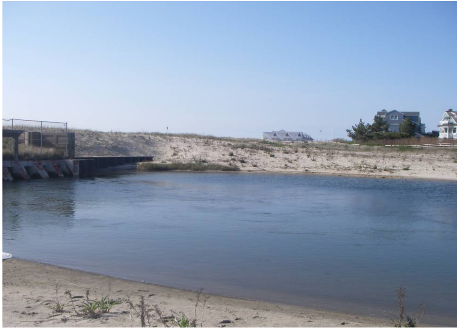
Photo 1: View facing southeast along shoreline of the first pond in the Wreck Pond watershed closest to the ocean. The outfall structure connected to the Atlantic Ocean is located to the left of the photo. Photo taken in 2008.
